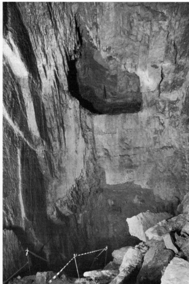
Looking north from the same camera position as picture to the left. The lower opening leads down to the canal tunnel. The upper opening extends over the canal tunnel. The mound of spoil in the foreground is to be removed.
